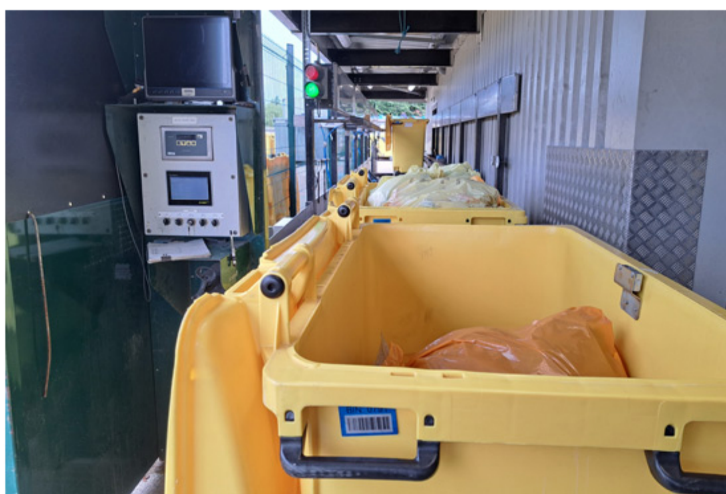
Yellow bins on the conveyor belt going into the incinerator
